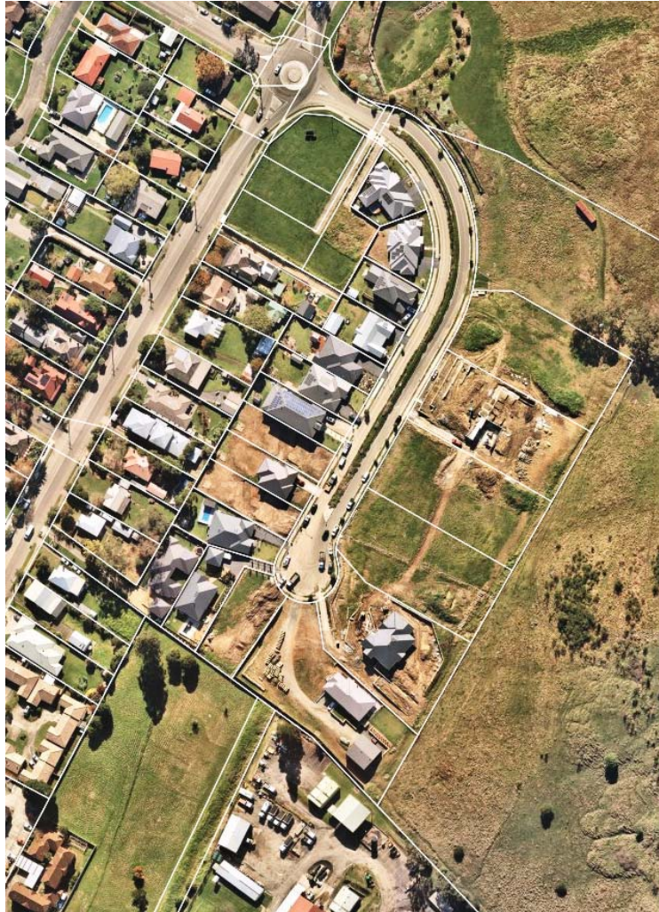
Aerial photograph of Eliza Place taken Tuesday 3 rd May 2022
